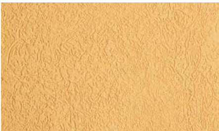
Rustic texture produced with Ceresit CT 35 mineral plaster, grain size 2.5 mm, obtained by floating with a plastic float in one direction
