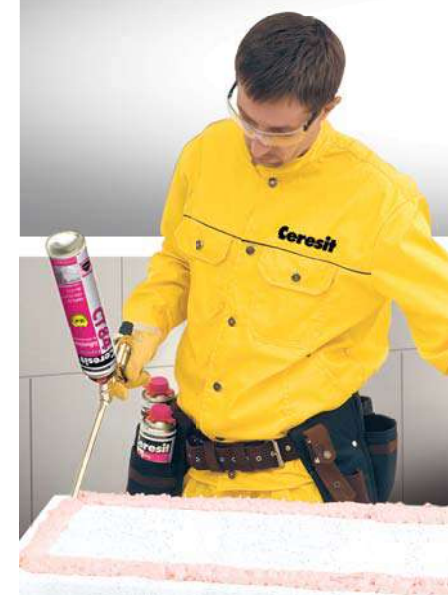
Fixing EPS board in thermal insulation system
