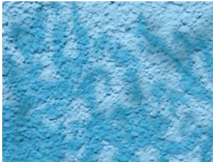
dirt gets into paint structure
