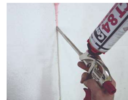
Filling in gaps between boards
